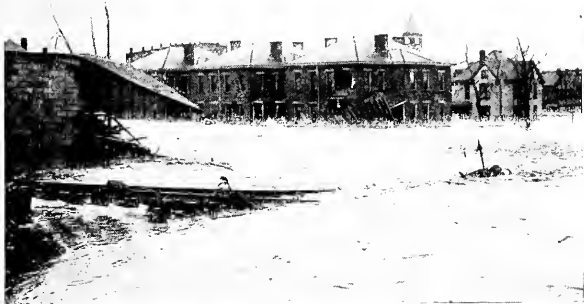
COLUMBUS: BRICK HOUSES BATTERED BY HEAVY DRIFTWOOD
